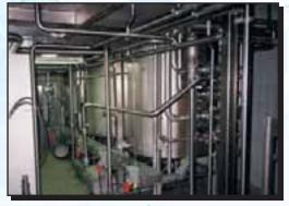
Leveltransmitters on CIP tanks
