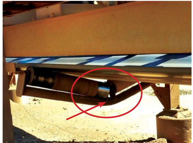
Idler Shell Collapse
